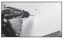
**Drill Actuator Holes.** Use a 3/16" drill bit to drill the three holes. (For aluminum boats, use 1/4-20 machine screws of an appropriate length instead of the screws supplied.)
